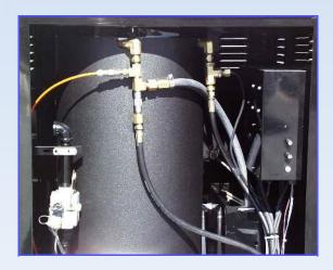
Gas Valve, Float Tank, Relief Valve, High Limit Switch, and Control Fuses are conveniently located behind the
