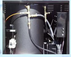
Gas Valve, Float Tank, Relief Valve, High Limit Switch, and Control Fuses are conveniently located behind the Upper Access Door.
